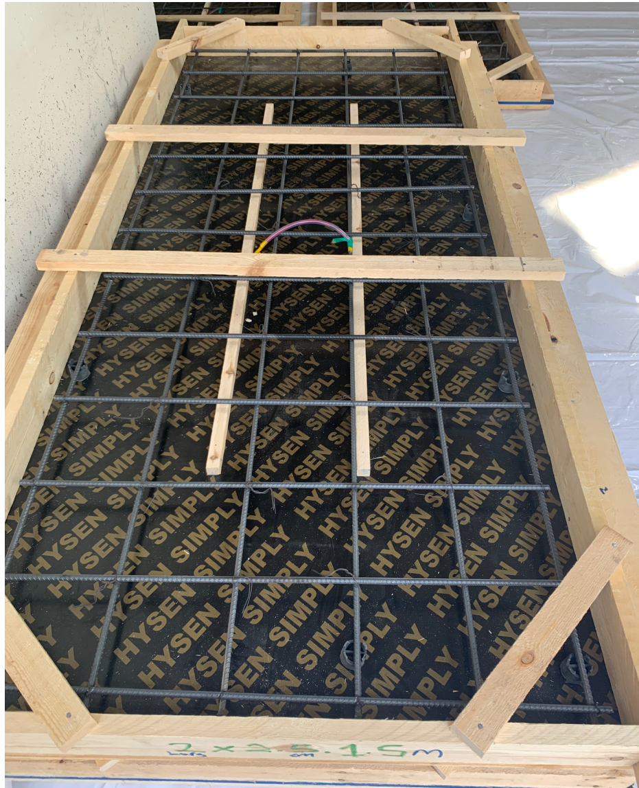
Figure 3.9 Slab Formwork and Reinforcement
